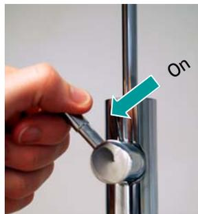
2. Turn on the dispenser tap to release the pressure in the system. Leave the tap in the 'on' position.
