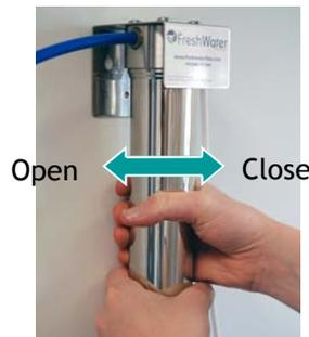
3. Leave the housing assembly on the bracket. Firmly grip the sump with both hands and turn to the left to release the seal. The sump of the filter will be full of water so position the bowl carefully to catch the residual water.
